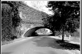
Yesler Trolley Bridge - 1930
